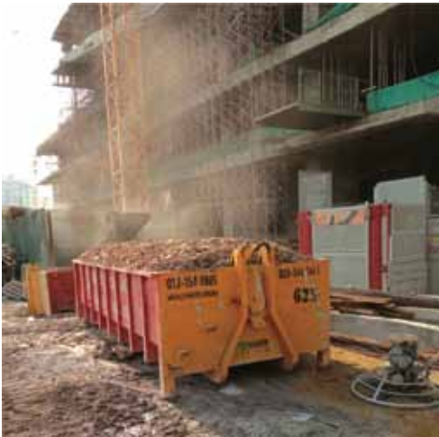
RORO bin at one of our development sites
